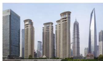
Tomson Riviera Apartment Towers Shanghai, China
